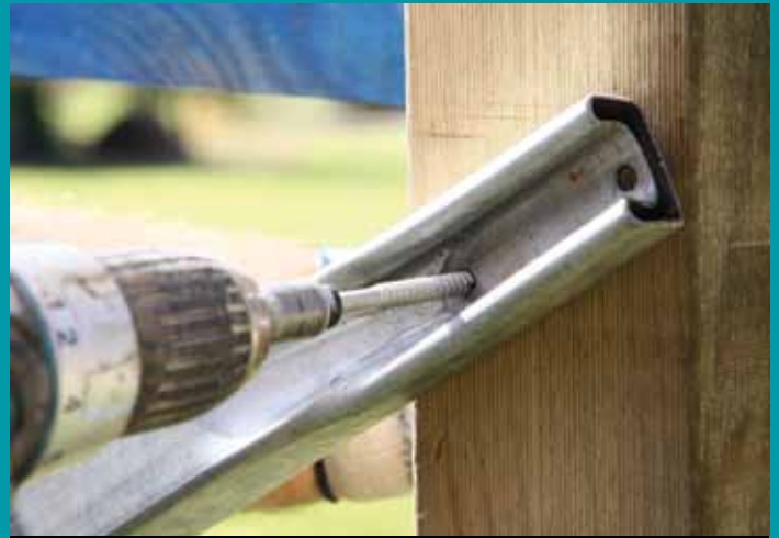
Affixing Uni-Brace® to a timber post.
