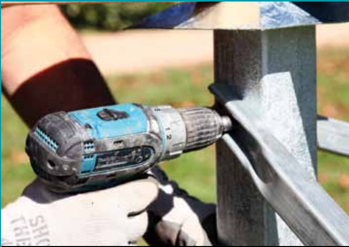
Screw fixing Uni-Brace® to top of post.
